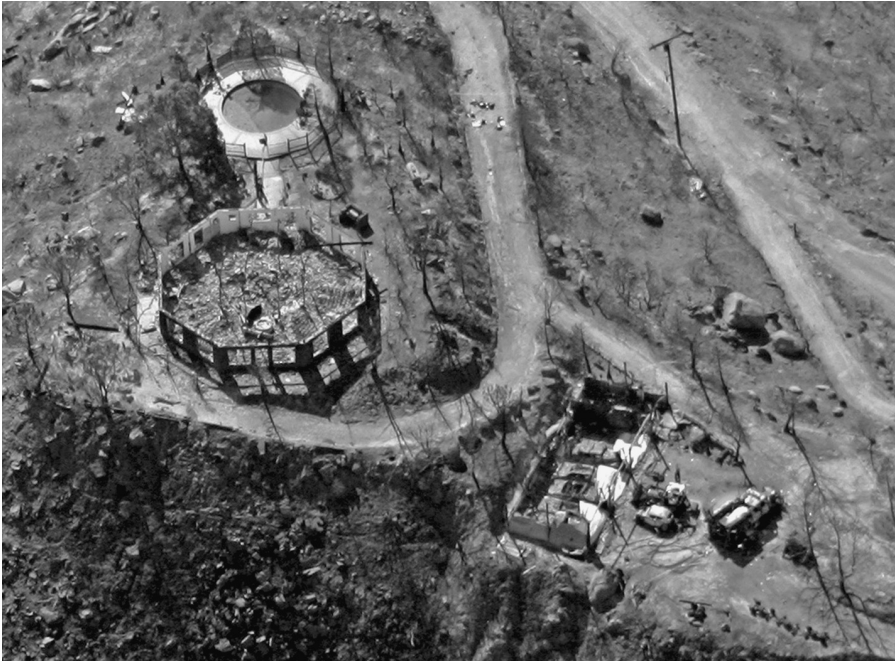
Figure 11.1 The Octagon House after the Esperanza Fire. Engine 57 is in the lower right corner. (Photo courtesy of AP's Reed Saxon.)
