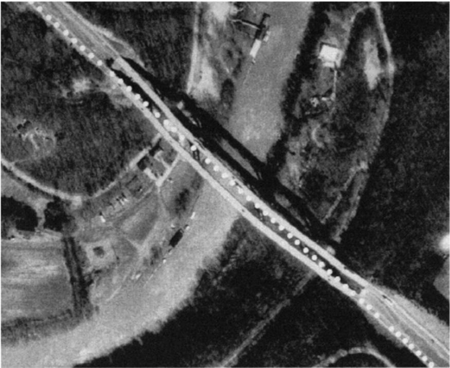
Figure 5-10. Displacement of bridge spans in orthophoto due to altitude differences.
